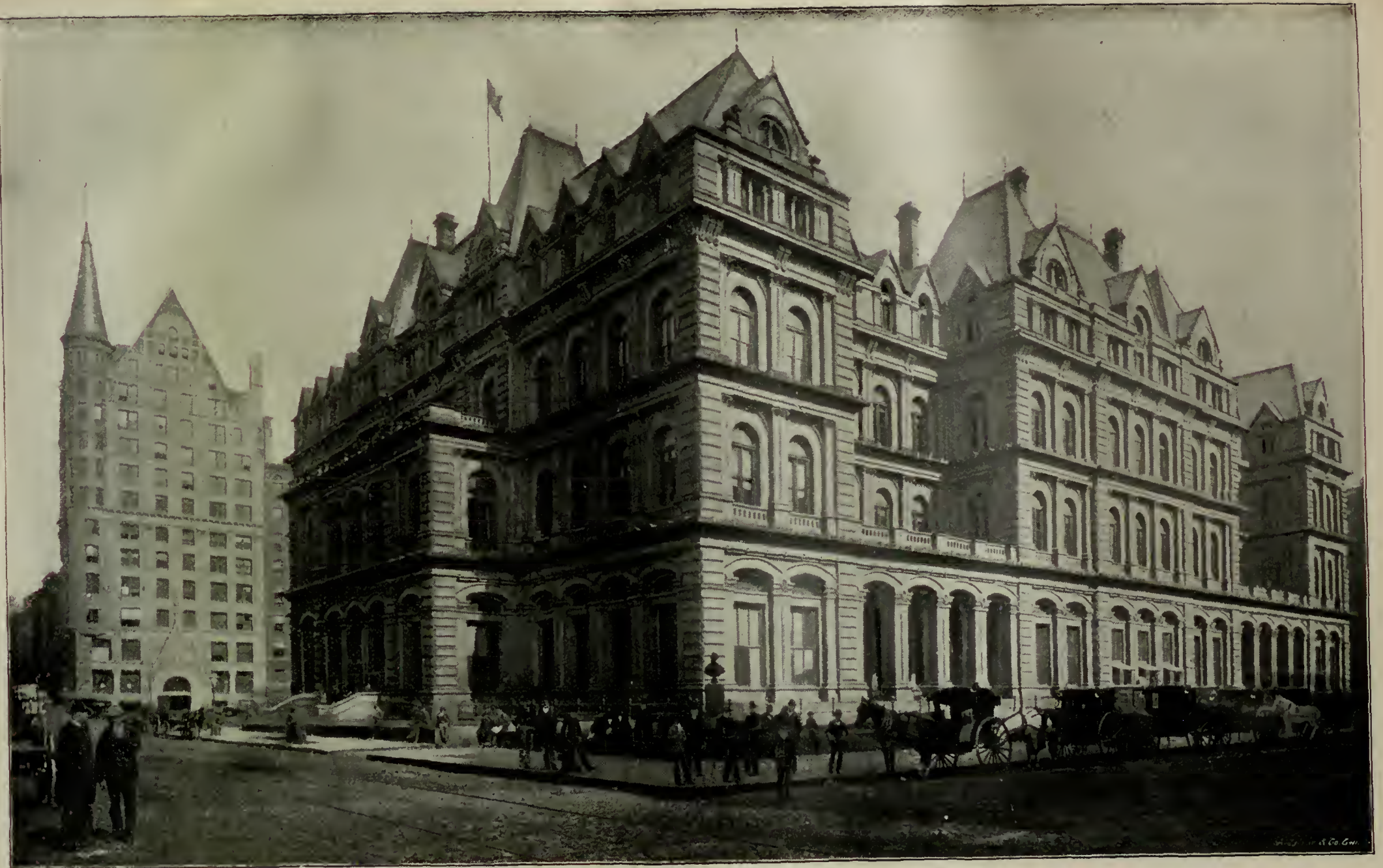
OWINGS BLOCK AND GOVERNMENT BUILDING.
